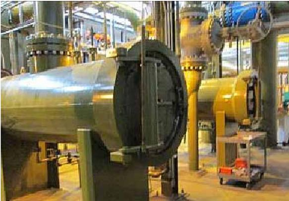
*Pentair dust filters for removing desiccant fines and solid contaminants upstream of the cryogenic plant*
